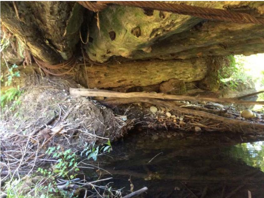
Left Bank Abutment when facing downstream
