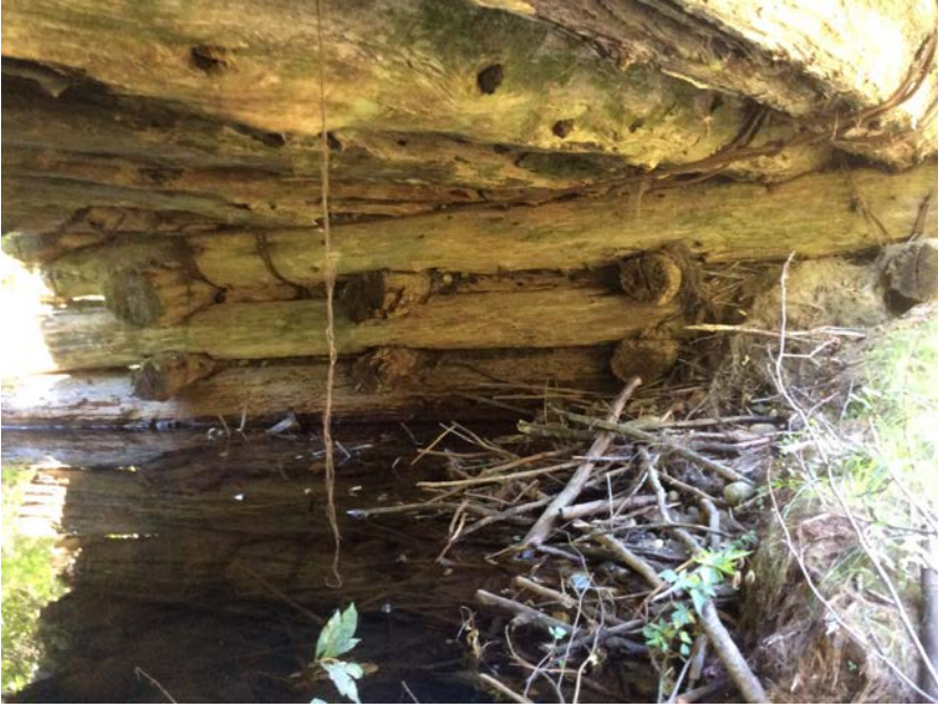
Right Bank Abutment when facing downstream
