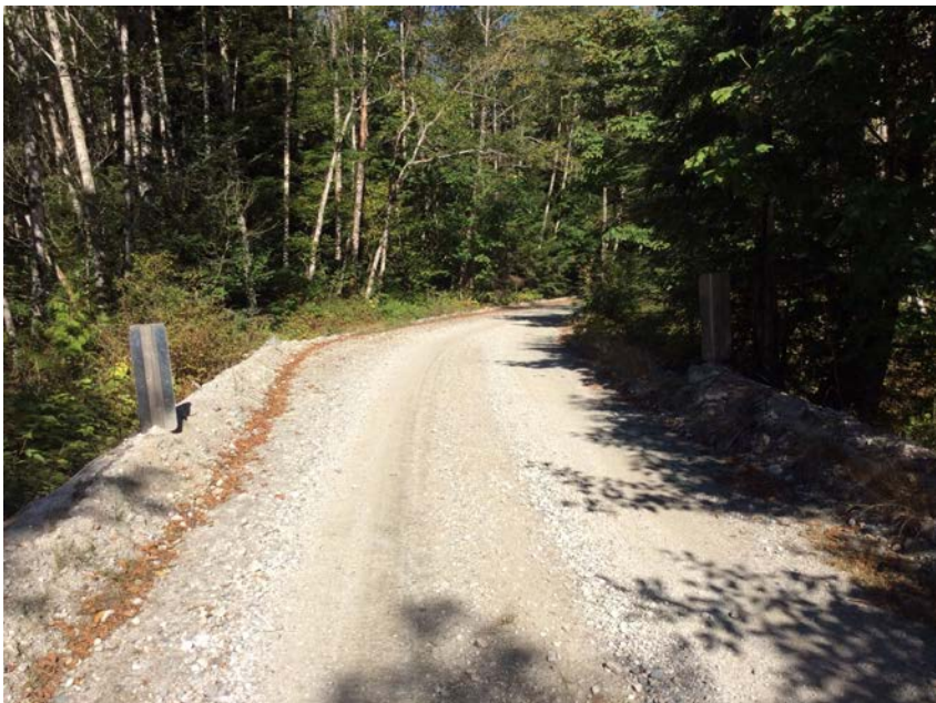
Right approach viewed from bridge
